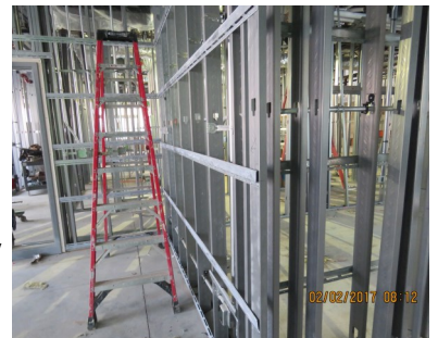
Proper RC Installation
